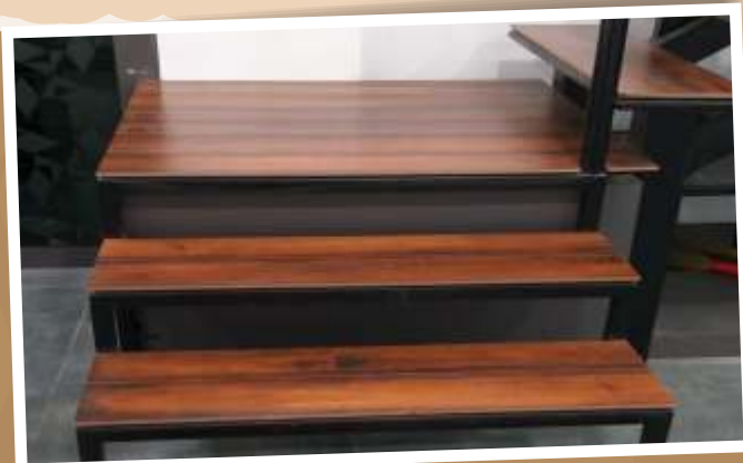
Flooring used in stair case
