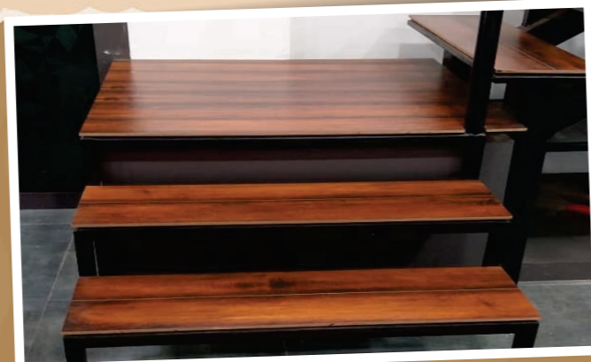
Flooring used in stair case
