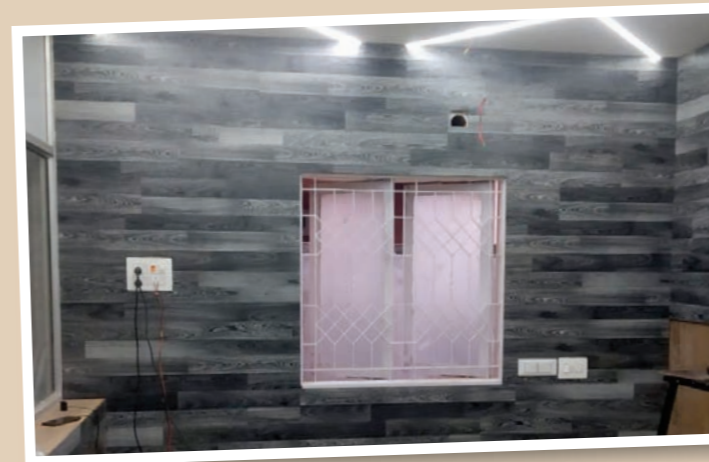
Flooring used in Wall Paneling
