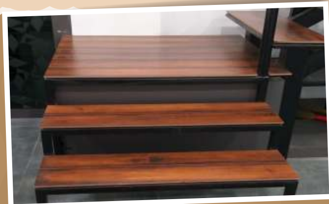
Flooring used in stair case
