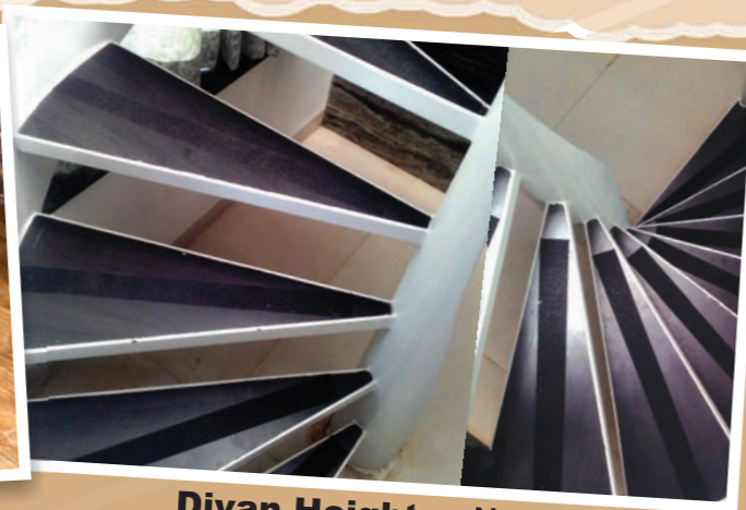
Divan Heights - Nasik Flooring used in stair case
