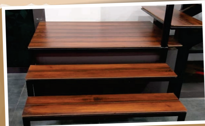
Flooring used in stair case
