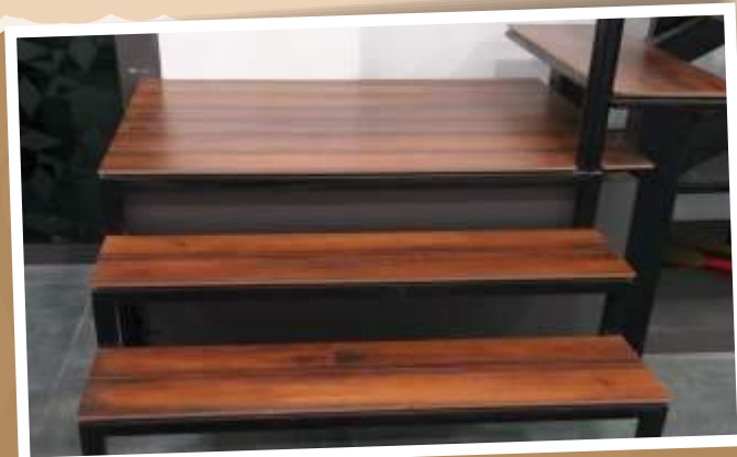
Flooring used in stair case
