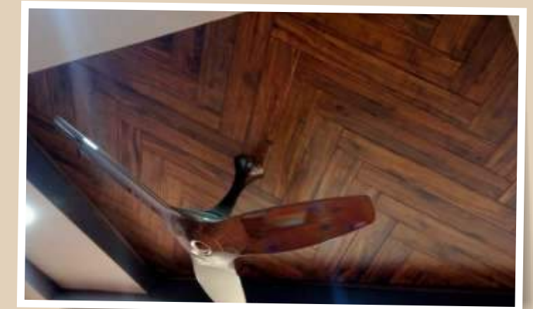
Flooring used in ceiling
